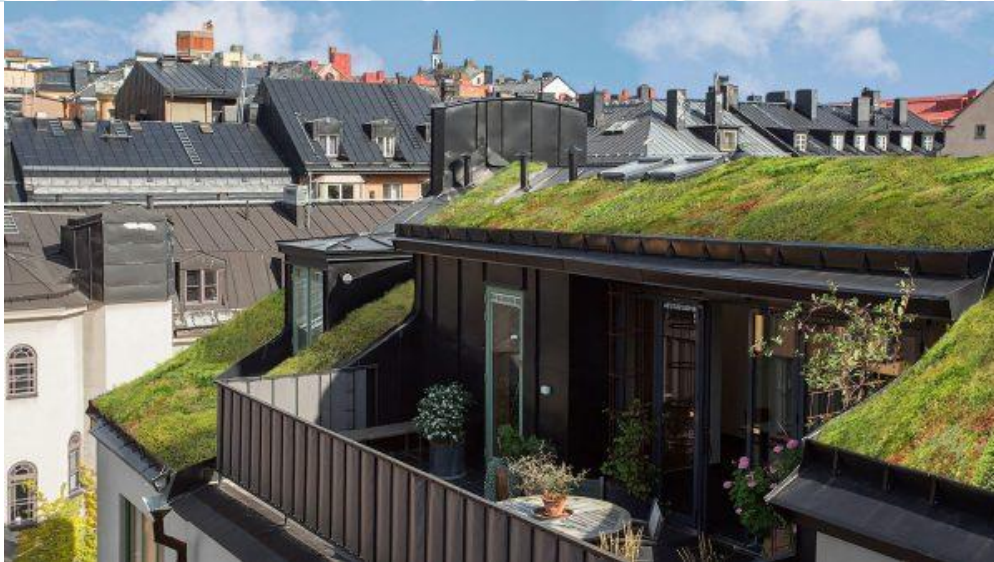
Picture 7: Green roof on apartment in Vienna, Austria (source: plantika.at )
