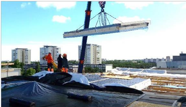
Picture 6: Installation of prefabricated panels on an apartment building's roof in Estonia (source: Kodi et al., 2024 )
