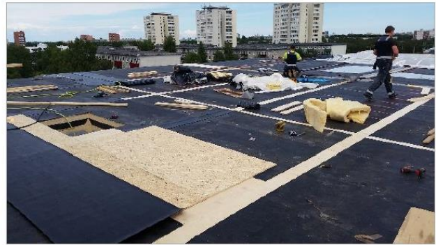
Picture 6: Installation of prefabricated panels on an apartment building's roof in Estonia (source: Kodi et al., 2024 )
